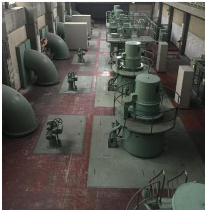
The second step is sending the collected water to reclamation centers. To maintain the sewerage system at a recommended depth it is necessary to use **pumping stations**. Pumps also help prevent floods by pumping large amounts of water in the event of heavy rainfall. So the purpose of pumps is to elevate the water level to continue the natural flow through gravity.
