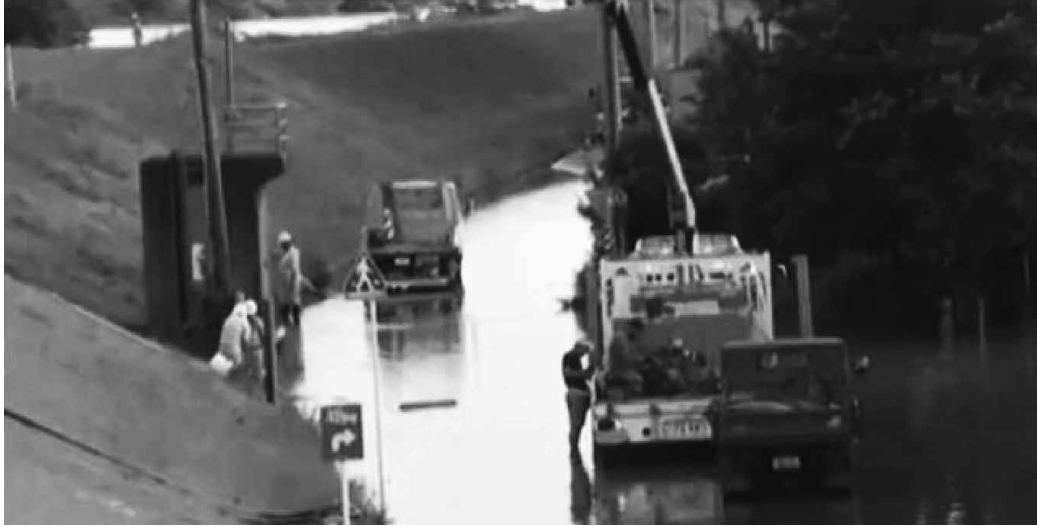
Figure 6 Photo showing that an area behind dike suffered from water logging
